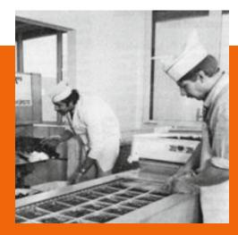
In 1984, a meat processing plant in Nuremberg, Germany, used a cryogenic tunnel freezer from Messer to cool pre-cooked sausages and then pack them in airtight packaging. This gave the products a shelf life of up to four months.
