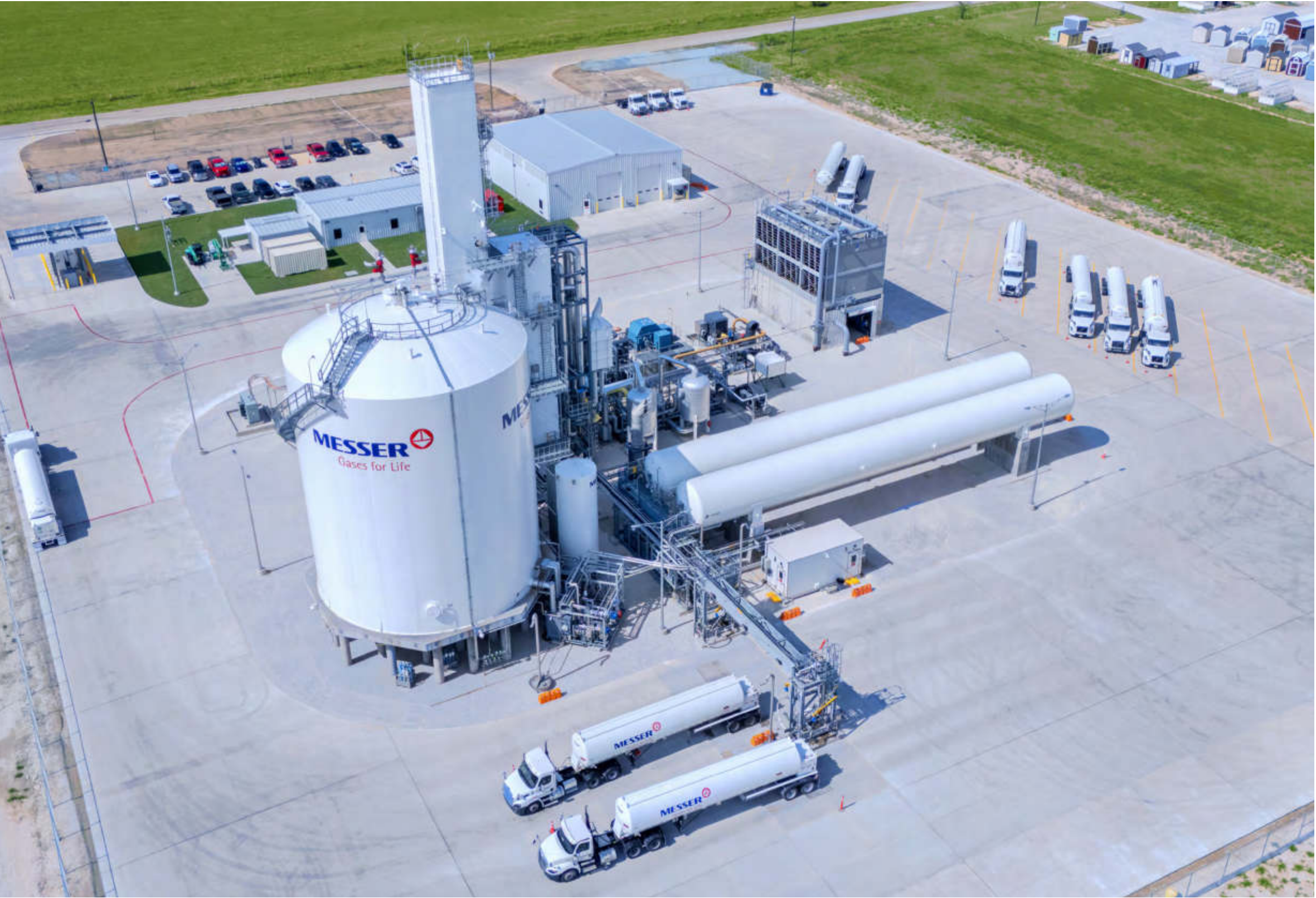
The air separation unit in McGregor, TX, operates substantially off energy supplied from an onsite solar panel array.
