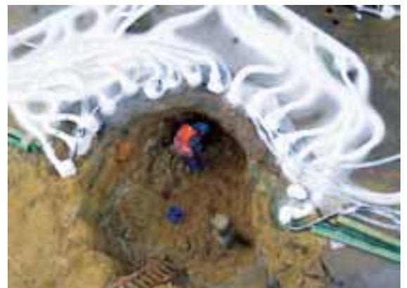
*A bird's-eye view of the excavation, clearly showing how the individual hoses feed the liquid nitrogen into the soil.*
