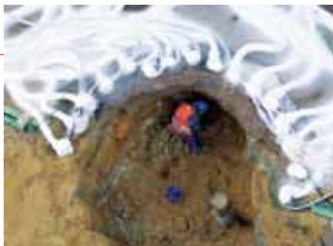
*Liquid nitrogen is pumped into the ground through a network of hoses and pipes.*
