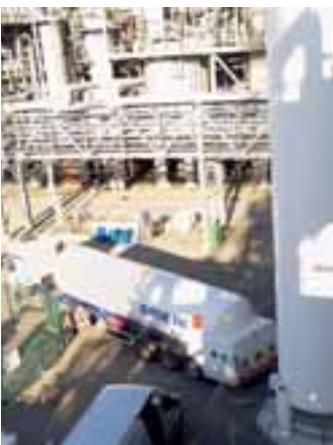
*The liquid nitrogen is transported to the site in large tankers and fed into on-site tanks.*
