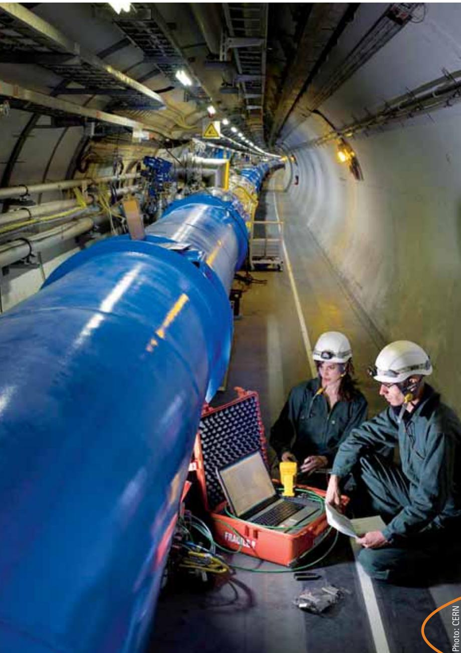
*A team of CERN engineers checks the electronics of the cryogenic instruments on a superconducting magnet.*
