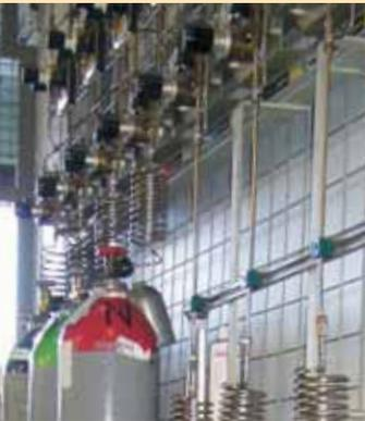
Central supply unit for high-purity gases.
