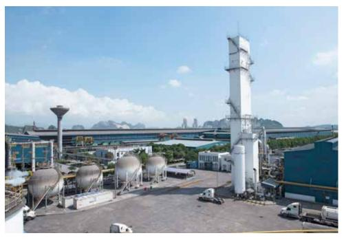
The air separation unit in the north of Vietnam supplies steel producer Hoa Phat Steel.
