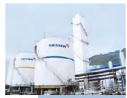
The new air separation units have a total capacity of 35,000 standar cubic metres per hour.
