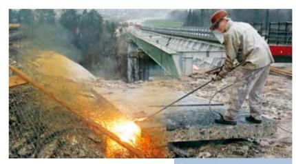
Concrete cutting with oxygen lances generates temperatures of up to 2 500 degrees centigrade
