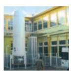
Kuhnke in Romania uses liquid nitrogen for inerting during the soldering of electronic components.
