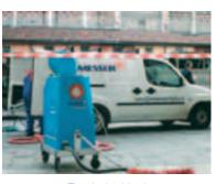
The dry ice blasting process from Messer was used to remove chewing aum from the cobblestones in the historical town center of Ferrara.
