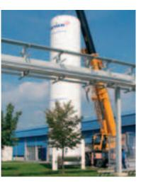
A central gas supply for air gases and specialty gases was installed at the leading Slovenian pharmaceutical company Lek.
