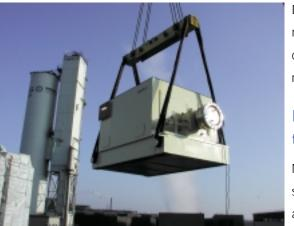
Delivery of the drive motor for the air separation plant in Dillingen
