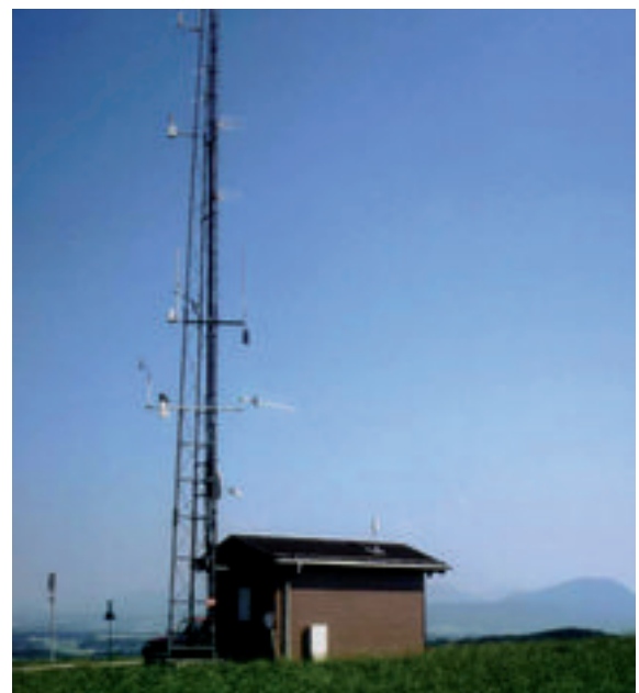
Air quality monitoring high in the mountains
